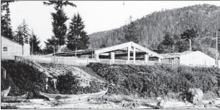
Figure 9. House lots 5 to 8. House 5, the first house to show in a photograph, is seen in part on the left in this detail of the Dosseter photo. It has a new façade of sawn lumber and a glazed window mounted high on the wall to prevent shooting inhabitants through the window during raids. Fenced gardens flank the foreshore of the midden. A square tower is under construction beside this house which is probably a bell tower for the school that was built about this time in this location.
