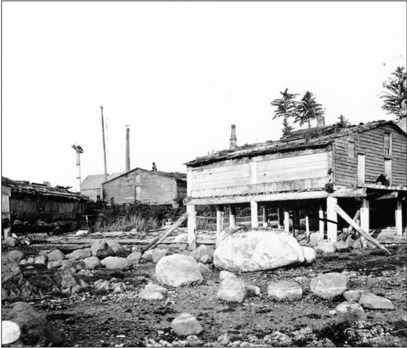
Figure 30. The "Beyond Creek" section of the village where some of the houses were built on log piers over the intertidal zone. Dossetter, AMNH 1881
