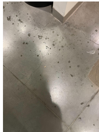
Figure 4. Cement floor in UBC LIFE building bathroom.
