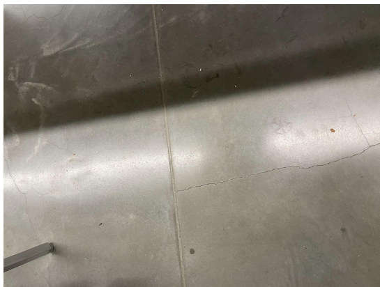
Figure 3. Cement floor in UBC LIFE building cafeteria.
