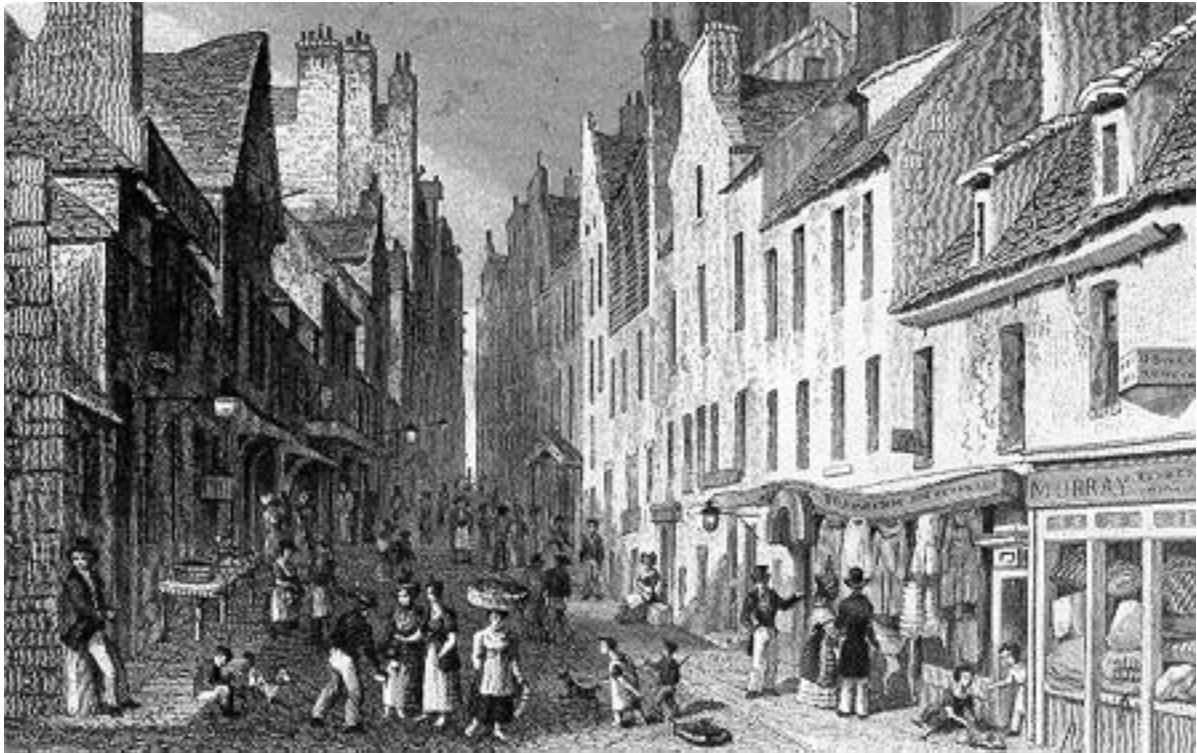
Figure 6: St Mary's Wynd, from the Pleasance, drawn by T.H. Shepherd, used with permission of the National Galleries of Scotland.
