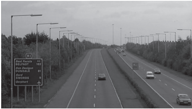
Figure 5: On the “straight” path—Git and Bunny drive off down the highway toward Dublin Airport
