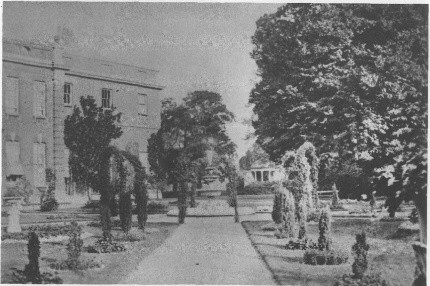
Figure 8. An exterior view of Gordon House.
