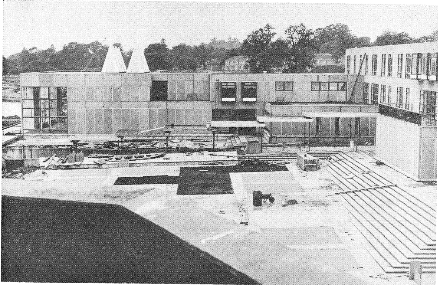
FIG. 3. A residential college of the University of York. The CLASP Mark IV system was used throughout the University for academic and residential buildings.
