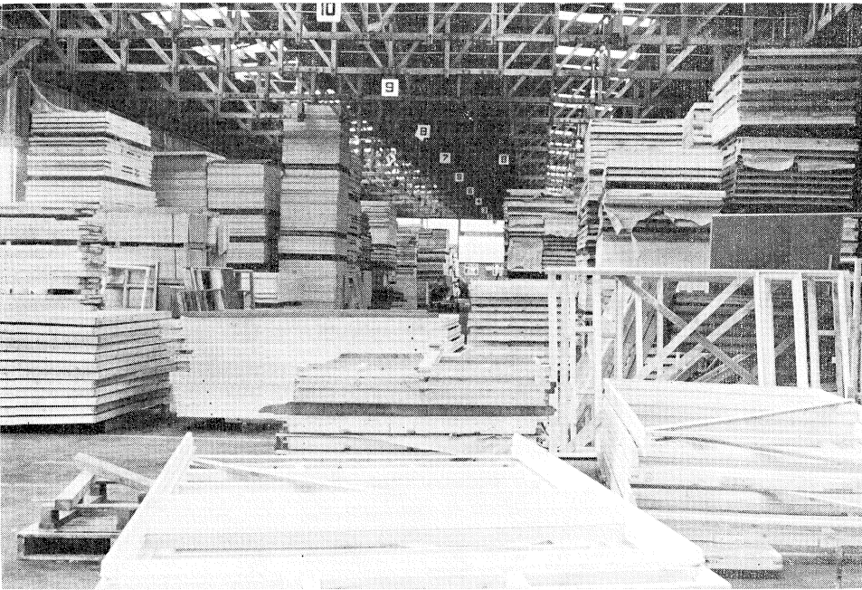
FIG. 2. Stock pile of timber wall components of the DERWENT system.
