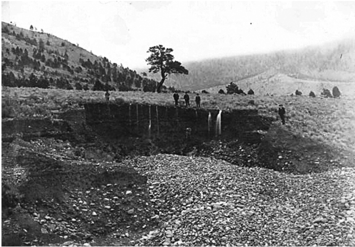
Figure 3. Ground sluicing above Lillooet. Source: Phair collection.
