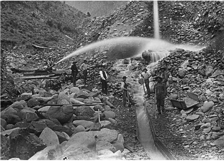
Figure 4. Hydraulic mining at the “Old Bridge” site. Source: Phair collection.
