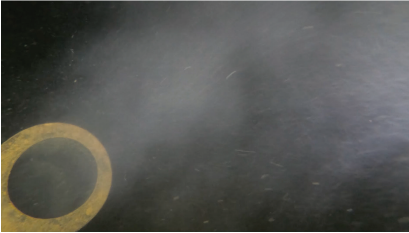
Figure 3. One of four diffusers discharging MPMC effluent 45 and 50 metres below surface of Quesnel Lake (screenshot from video at www.ccql.ca ).
