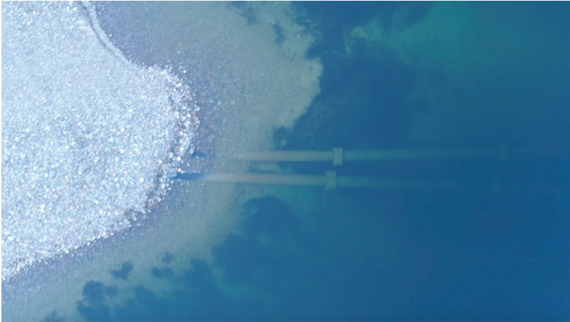
Figure 1. Two 24-inch MPMC effluent pipelines entering Quesnel Lake near mouth of Hazeltine Creek (screenshot from video at www.ccql.ca ).
