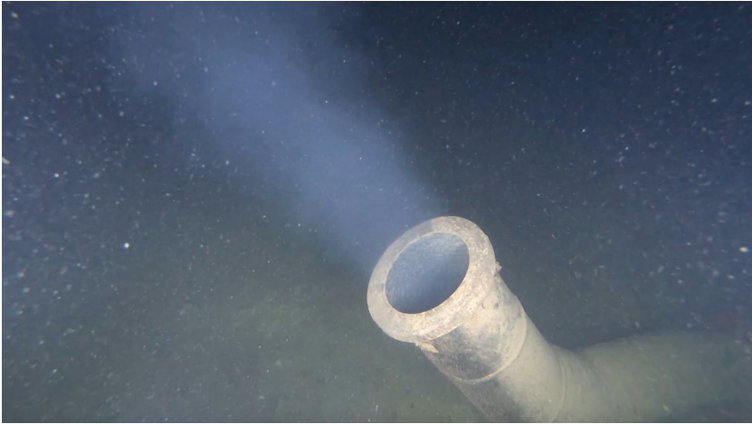
Figure 2. One of four diffusers discharging up to 10 million cubic metres annually of untreated MPMC effluent into Quesnel Lake (screenshot from video at www.ccql.ca ).
