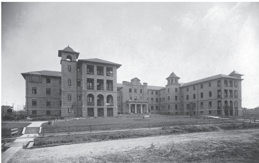
Figure 13. Vancouver General Hospital in Fairview under construction, 1905. Source: City of Vancouver Archives (hereafter CVA), AM336-S3-2-, CVA 677-506.
