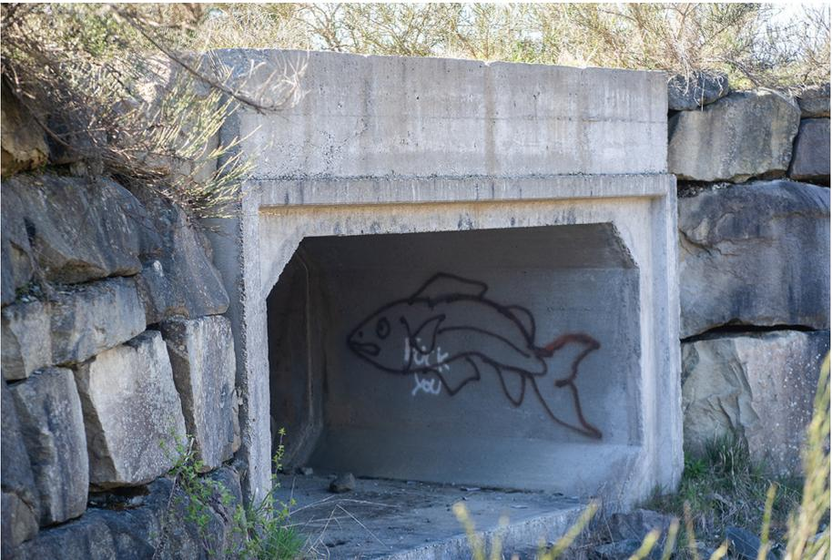
Figure 4. Concrete Culvert. Photo by Brette Little.
