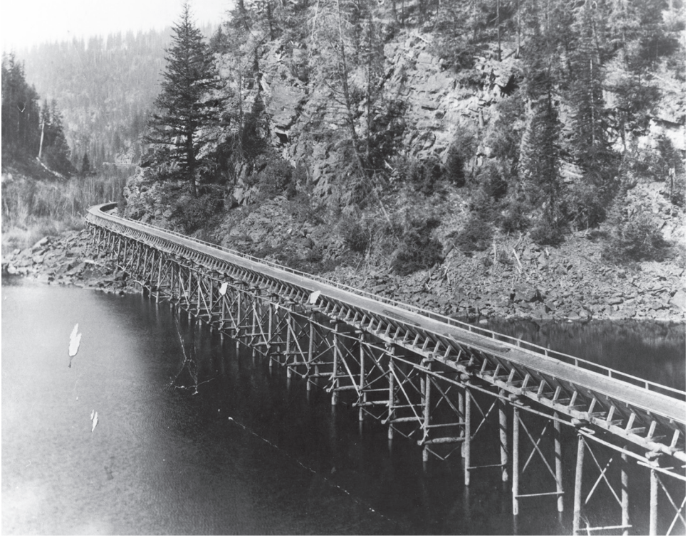
Figure 3. BC Spruce Mills flume carrying logs, ca. 1925. The company relied on an extensive flume system to move logs to the mill pond in Lumberton. Source: Columbia Basin Institute of Regional History, image 0008.0008.
