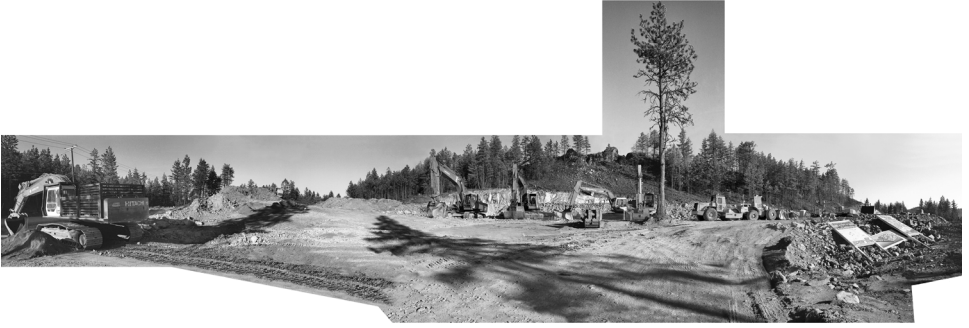
Preparing roads, future entrance to Panorama Peaks with remaining lone tree, 2004.
