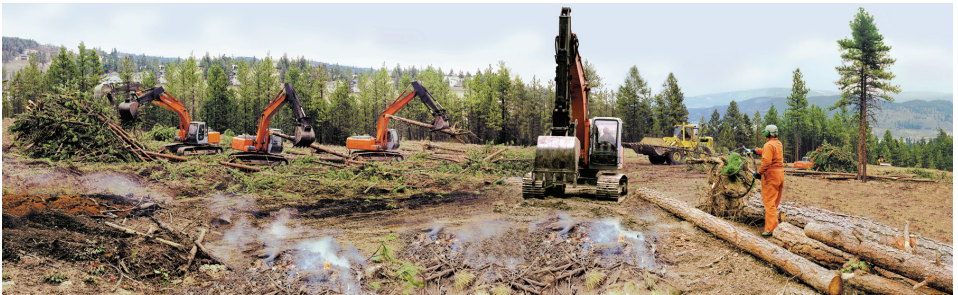
Clearing land for development in West Kelowna, 2000.
