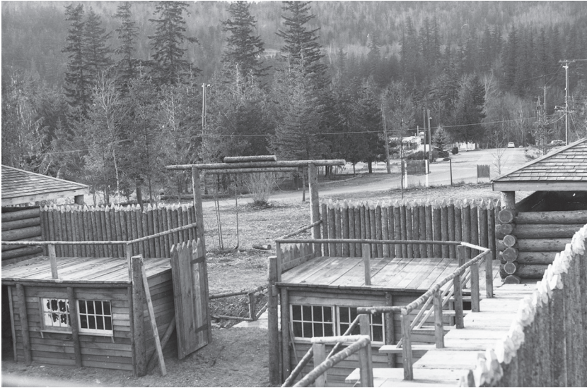
Figure 3. Frontier town built at Cultus Lake. Photograph courtesy Chilliwack Museum and Archives, 1999.029.004.087, 1960.
