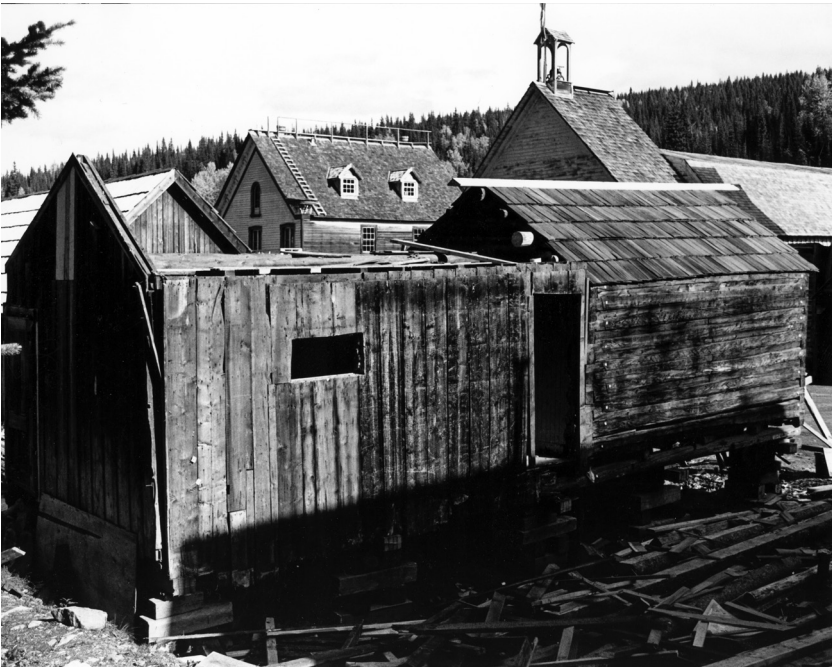
Figure 7. The Van Volkenburg cabin, during renovations, 1985, showing the vertical plank construction. Source : Barkerville Historic Town Photo Collection P2381.
