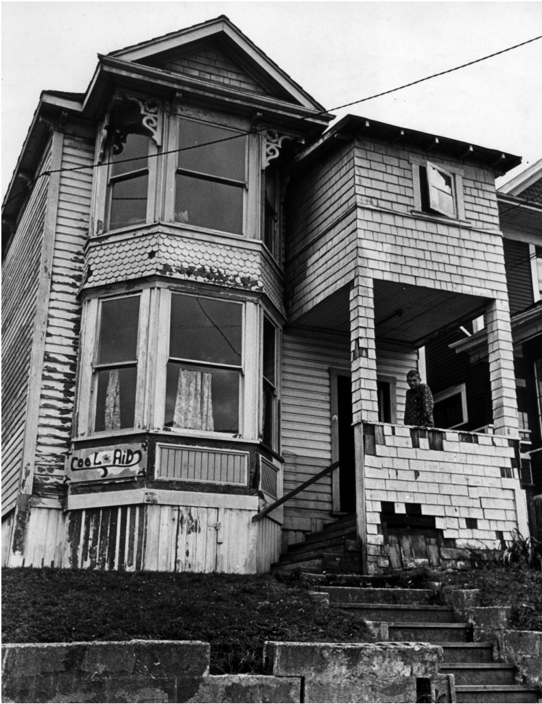
Figure 6. The Cool-Aid house at 1822 West 7th Avenue in Kitsilano in August 1968. Note the poor condition of the property that caused so much controversy at City Hall. Brian Kent/ Vancouver Sun .
