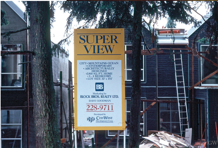
Fine new homes capturing super views – but often developed without concern for the environmental costs.
