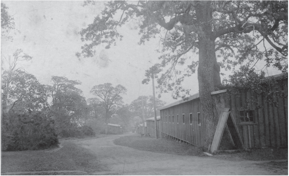
Figure 7. The BC Bantams' barracks at Beacon Hill Park, Victoria, ca. 1916. Note the rustic board-and-batten siding of these utilitarian structures. Source: Image 197909-38, Box 2, Container 000502-0001, courtesy of the Royal BC Museum, vca, Robert Ely Fonds.
