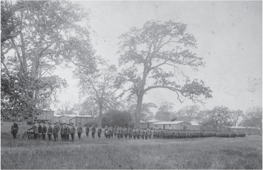
Figure 6. The BC Bantams in front of their barracks, beneath the Garry oaks at the north end of Beacon Hill Park, ca. 1916. The Daily Colonist describes the site as “under the spreading oaks facing Heywood Avenue at the entrance to the park.” Erection of the “hutments” began in February 1916, with some 400,000 feet of lumber donated by the City of Victoria, and a month later the camp was under construction by the Bantams themselves as well as by the Royal Canadian Engineers. Conceived as a single building, by late April 1916, the Colonist notes, the extensive camp included “barrack rooms, mess rooms, store buildings, hospital, orderly room, guardroom, etc.” Separate tents served as officers’ quarters. Source: Image 197909-38, Box 2, Container 000502-0001 courtesy of the Royal BC Museum, BCA, Robert Ely Fonds.
