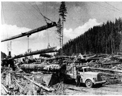
Logging Process, Yarding & Loading, O'Brien Logging Company: logs are "yarded" to a general point and loaded on waiting trucks for transportation to tide water. Special Collections, UBC Library, MacMillan Bloedel Limited Photograph Collection, Box 17, BC1930/262.
