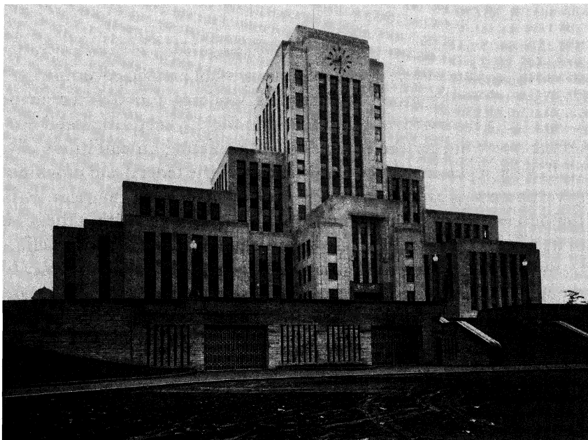
Figure 10: City Hall from the north, 1936. Note the podium and slit windows. (Vancouver Public Library, Special Collections, VPL 4688)
