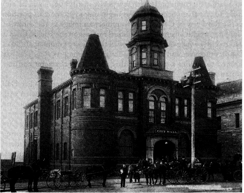
Figure 2: Old Vancouver City Hall in 1901. (City of Vancouver Archives, City P.47 N.40)
