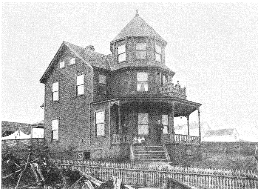
Turreted house, West End, ca. 1890
