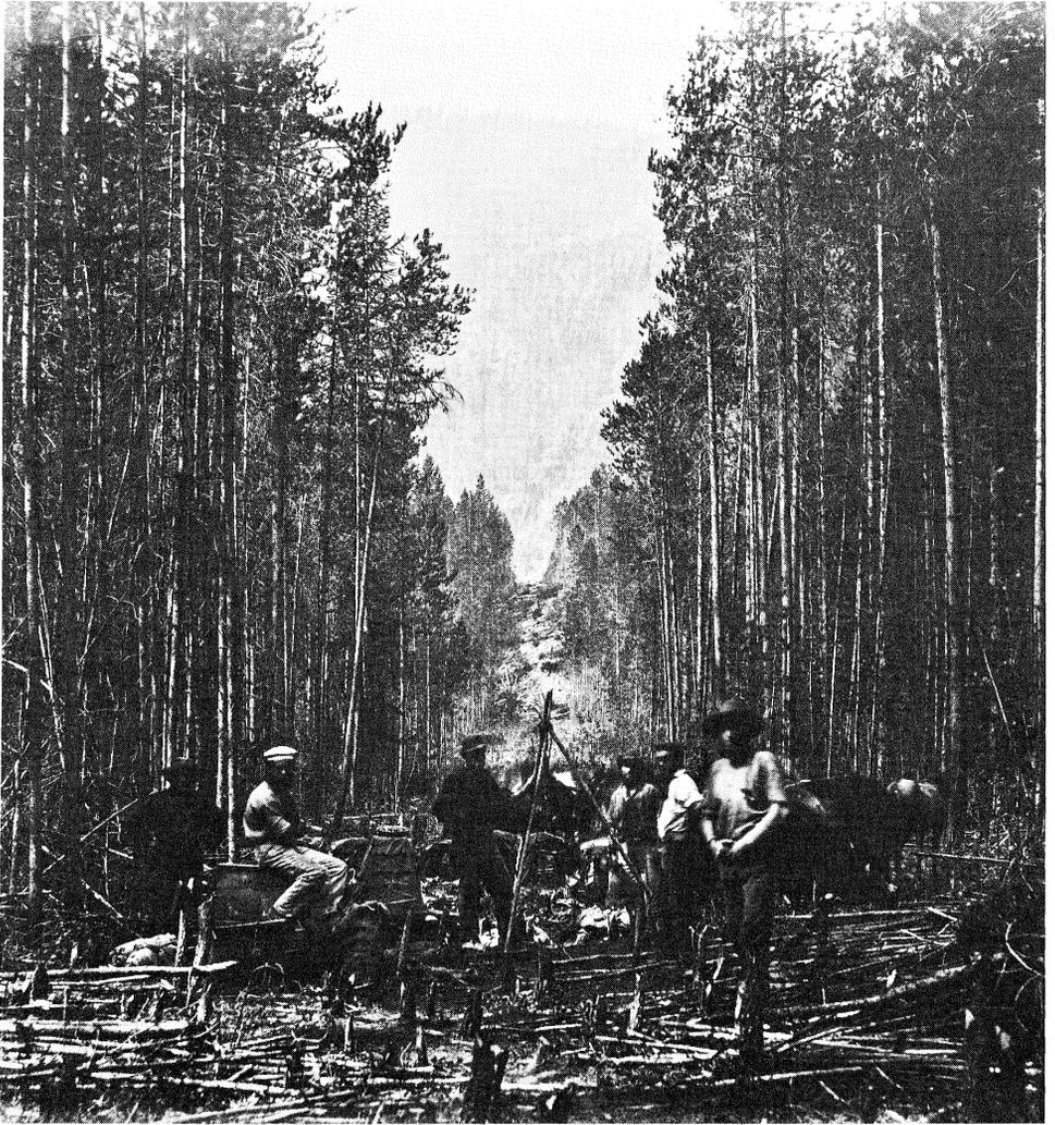
PLATE I. *Cutting on the 49th Parallel, on the right bank of the Mooyie River, looking west.* North American Boundary Commission, 1861. Photo: Royal Engineers (c-78979). Much of the photography on the earliest surveys was to show the nature of the work being done and the country through which the survey passed. This photo demonstrates clearly to the leaders at home how the boundary was marked and the densely-wooded terrain that was encountered.
