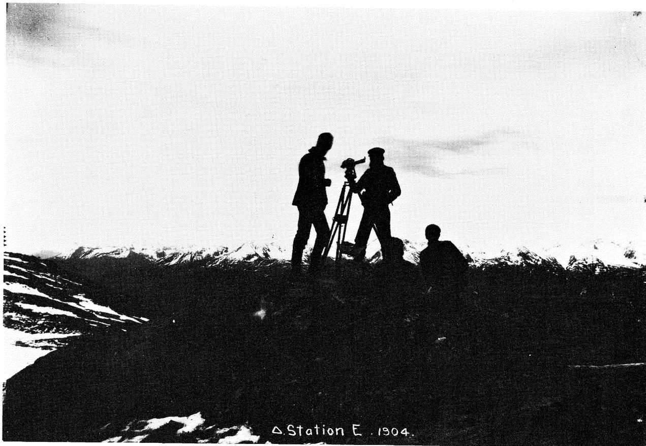
PLATE VI. *International Boundary Commission. Triangulation Station E, Chilkat River district, 1904* (PA-37740). This photograph by C. H. Bigger shows the surveyor's party on the summit of a mountain establishing the position of the camera station with a theodolite. The exact position was always noted in this way so that accurate maps could then be made from the photographs back in the survey offices.
