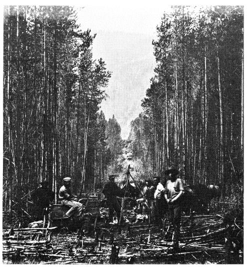
PLATE I. Cutting on the 49th Parallel, on the right bank of the Mooyie River, looking west. North American Boundary Commission, 1861. Photo: Royal Engineers (c-78979). Much of the photography on the earliest surveys was to show the nature of the work being done and the country through which the survey passed. This photo demonstrates clearly to the leaders at home how the boundary was marked and the densely-wooded terrain that was encountered.
