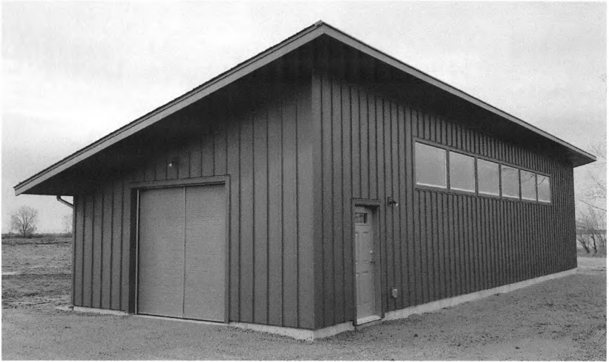
Figure 9. Musqueam Carving Shed. Exterior. Photo credit: Shelly Johnson.
